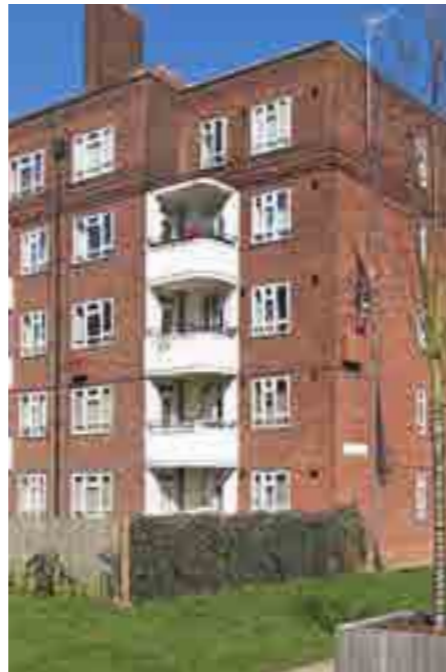
05 phase 4 corner balconies
