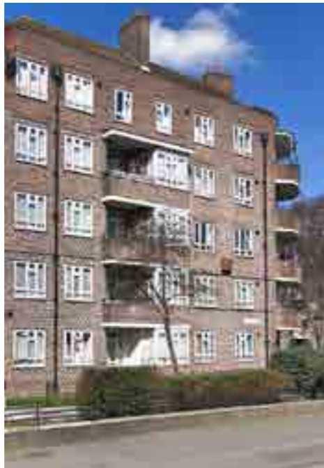
04 phase 6 stacked balconies
