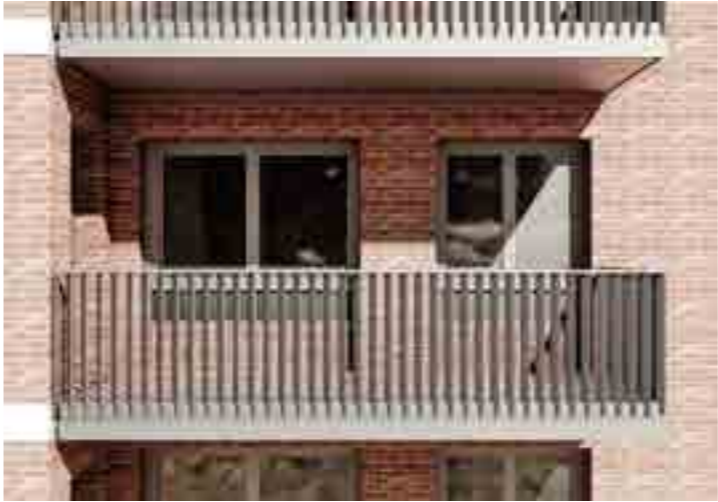
02a Woodberry Down balconies
